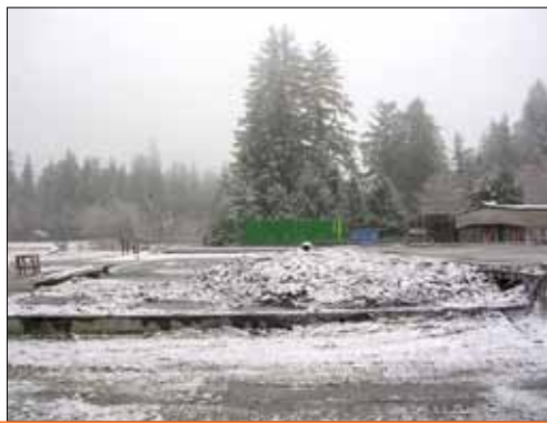
The site was already cleared and prepped for reconstruction within weeks of the fire. PHOTO BY KEVIN CHASE
