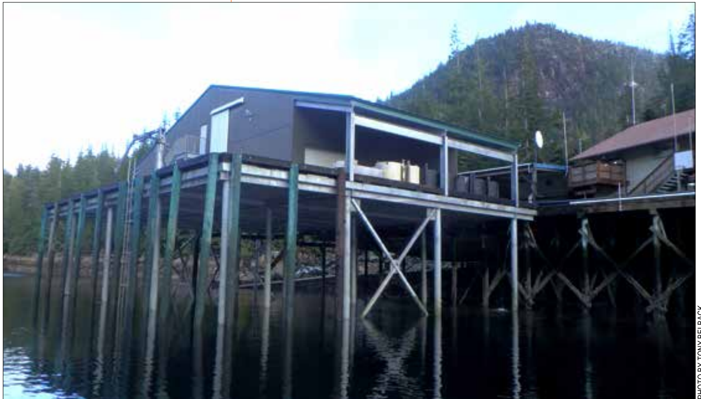
SSRAA built a new 6,000 square-foot concrete pad on steel pilings and an incubation facility at Burnett Inlet—one of two major planned projects.
